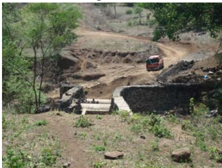
Looking down on the bridge from where the road goes now
